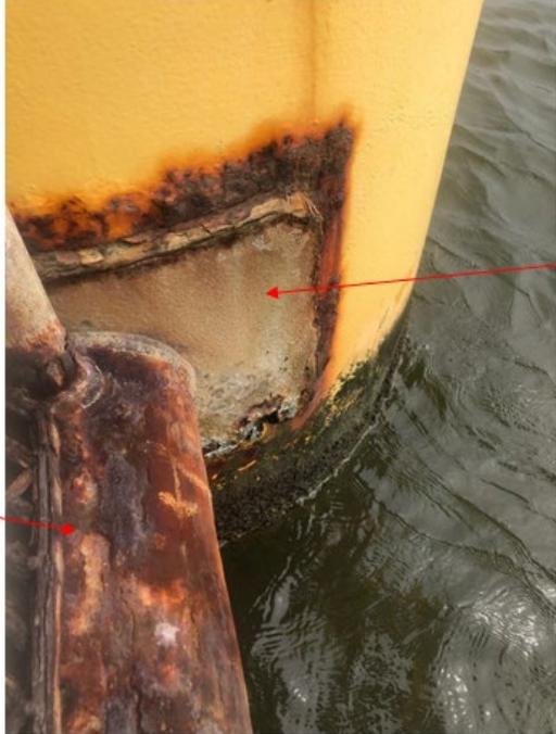
**Figure 15.** – Corrosion issues at the Calcasieu Pass SPIP boat landing doubler plates and support pipe beams
