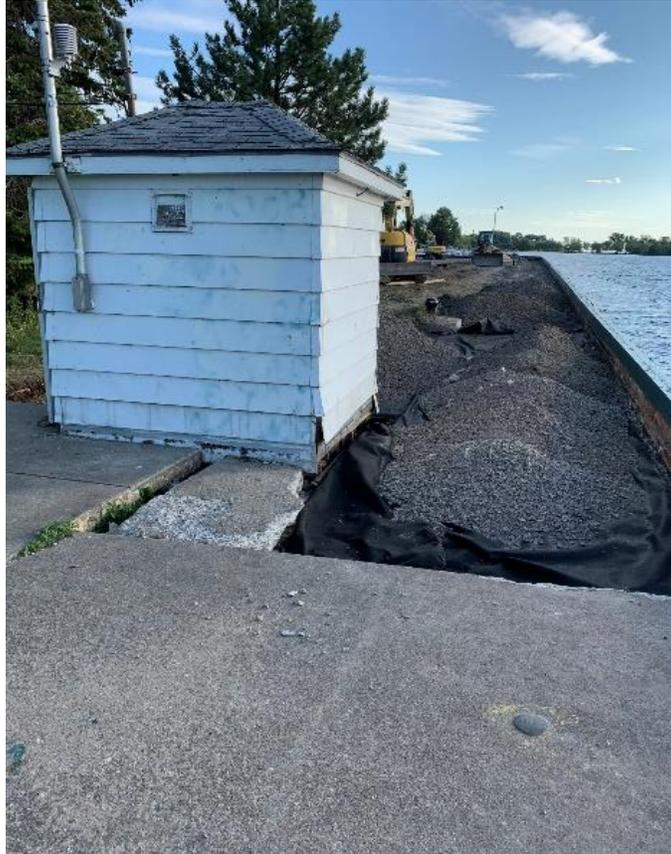
**Figure 12.** Ogdensburg, New York station and bulkhead erosion
