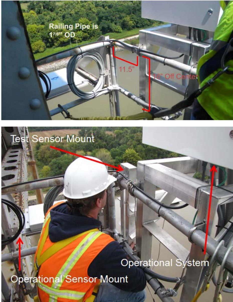
Figure 19. Sensor mounting.
