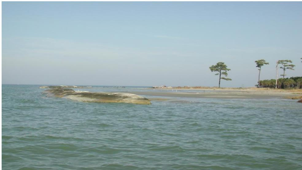
**Figure 2.** Geotextile tubes were placed on the northwest side of Barren Island by USACE to retain dredge material used to create new marsh uplands while providing a wave break for the eroding island.
