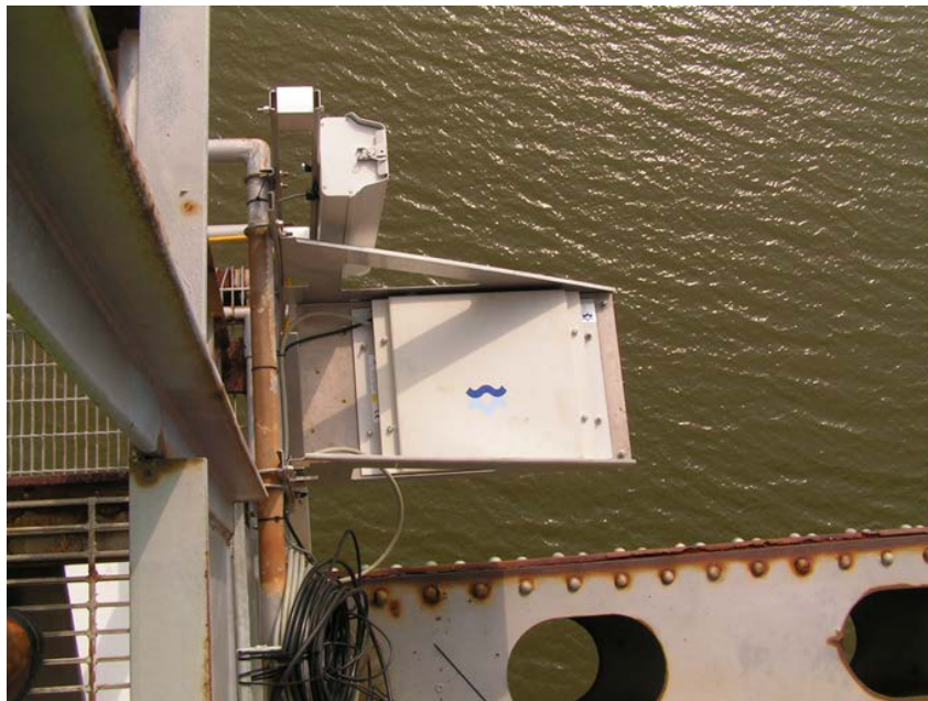
Figure 3-1. Top view of Reedy Point Bridge Miros mount.
