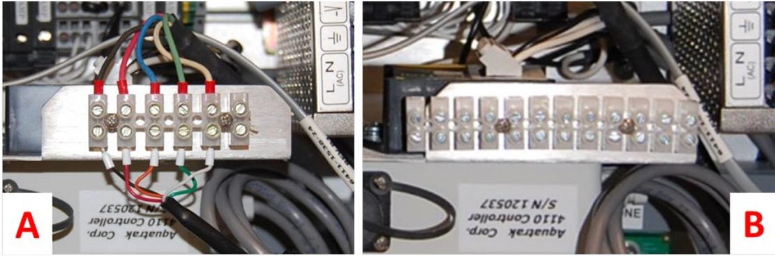
Figure 3-2. (A) The old terminal strip with the Aquatrak cable connected and (B) the new terminal strip.
