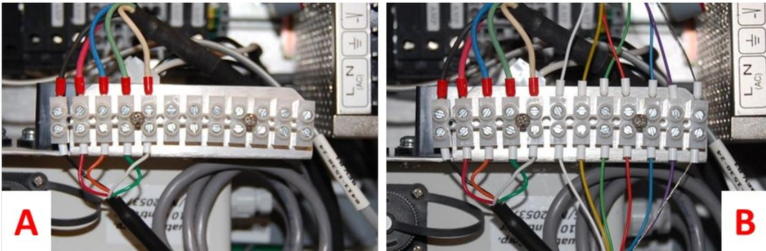
Figure 3-3. (A) New terminal strip with Aquatrak cable reconnect and (B) new terminal strip with Aquatrak and Greenspan cables connected.
