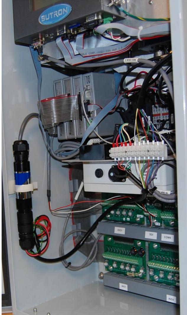
Figure 3-4. SDI-12 converted mounted on the wall of the enclosure.
